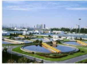
水处理厂: 污泥输送和抽取 Water treatment plant: sludge transport and extraction
