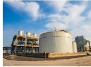
化工厂: 污水、污泥输送和抽取 Chemical plant: sewage, sludge transport and extraction
